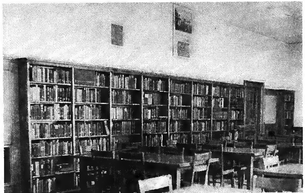
Typical speaker installation in library of Katonah High School. All classroom speakers are flush wall mounted with matching grille frames.
